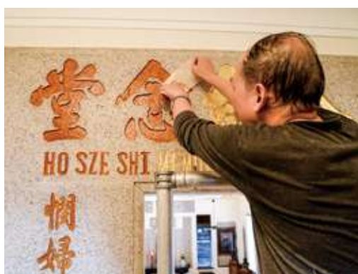
▲碑石的修復過程：清潔碑石表面，碑文髹金油，塗上金箔專用膠水，最後貼上金箔。 Process of conservation: apply cleaning agent on stone surface, re-colour inscription with gold paint, cover painted area with dedicated adhesive, complete by gilding gold leaves.
